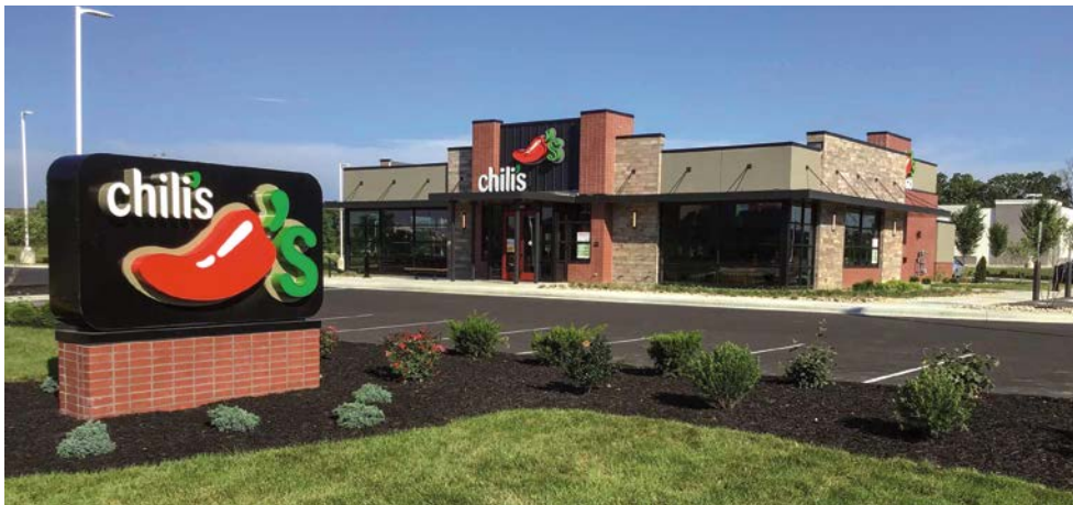
Above: A recently completed Chili's restaurant in Columbus, Ohio.
